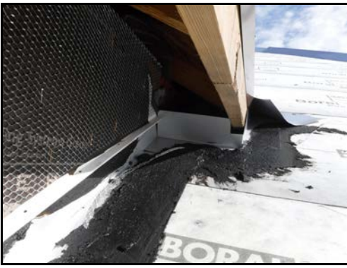
10. Metal flashing stop installed on right side of front entry soffit
