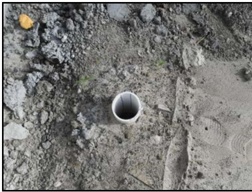
2. Missing sewer clean out
