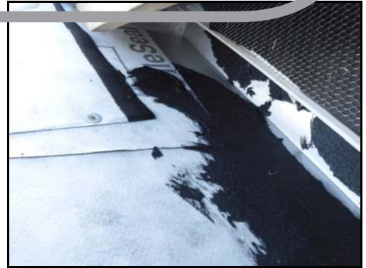
9. "L" flashing popped slightly on left side of front entry wall. No metal cap at top of soffit, like right side.
