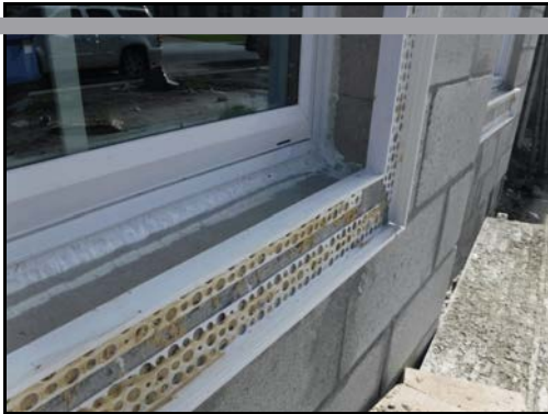
8. Make sure to maintain slope at stucco trim window sills
