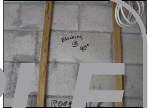
15. Not all blocking added at initial construction
