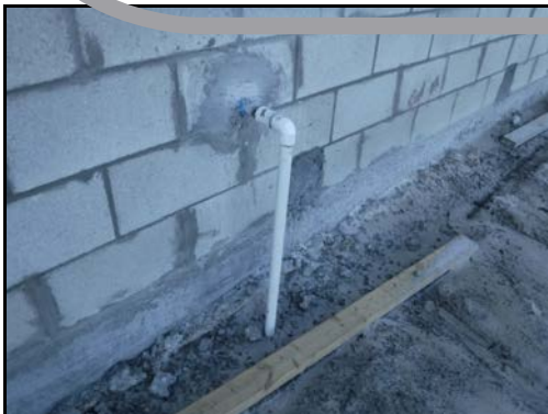
7. Water shut off valve to be installed later?
