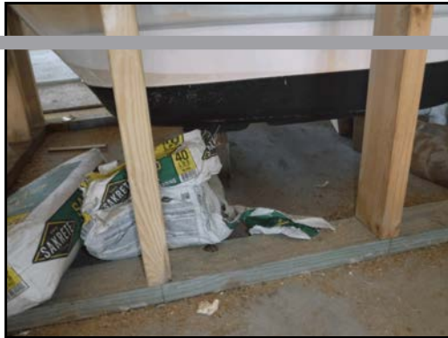
26. Master tub currently supported by wood blocks
