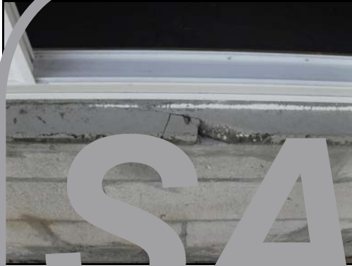
4. Damage to concrete window sill
