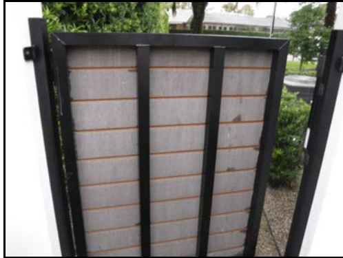
5. Latches to pool area do not self close.
