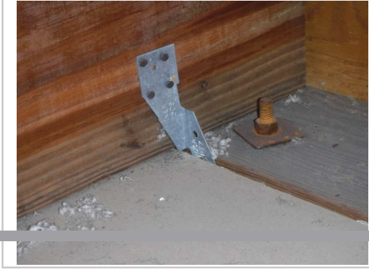
Roof to wall attachment - Clips
